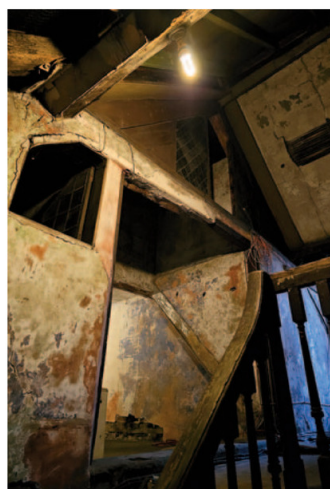
Top left: Exposed timber frame showing historic roofline
