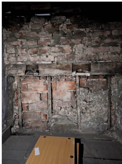
Top left: Exposed timber frame showing historic roofline
